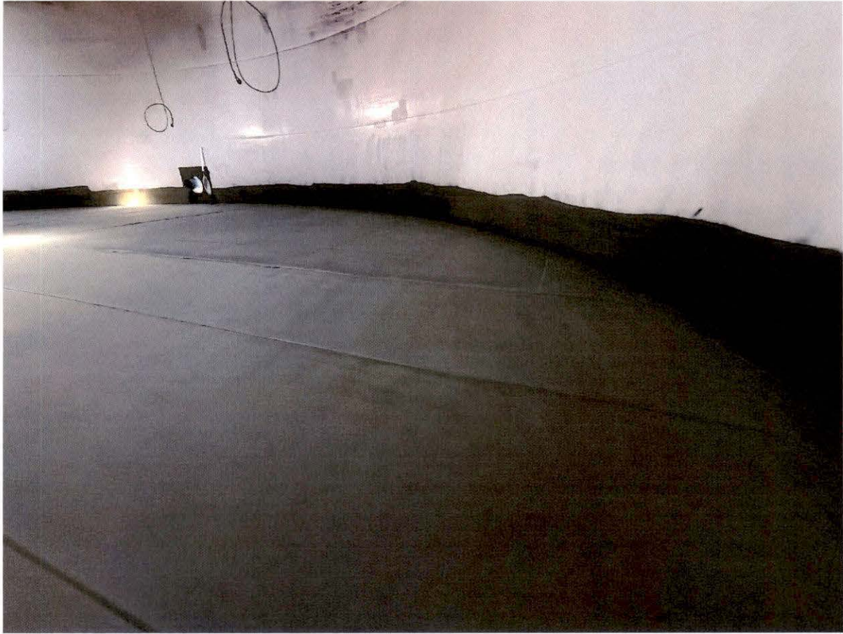
June 1, 2026 – Interior coating – First coat
