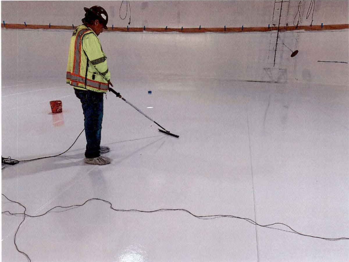
June 5, 2026 –Interior coating – Final coat & spark test
