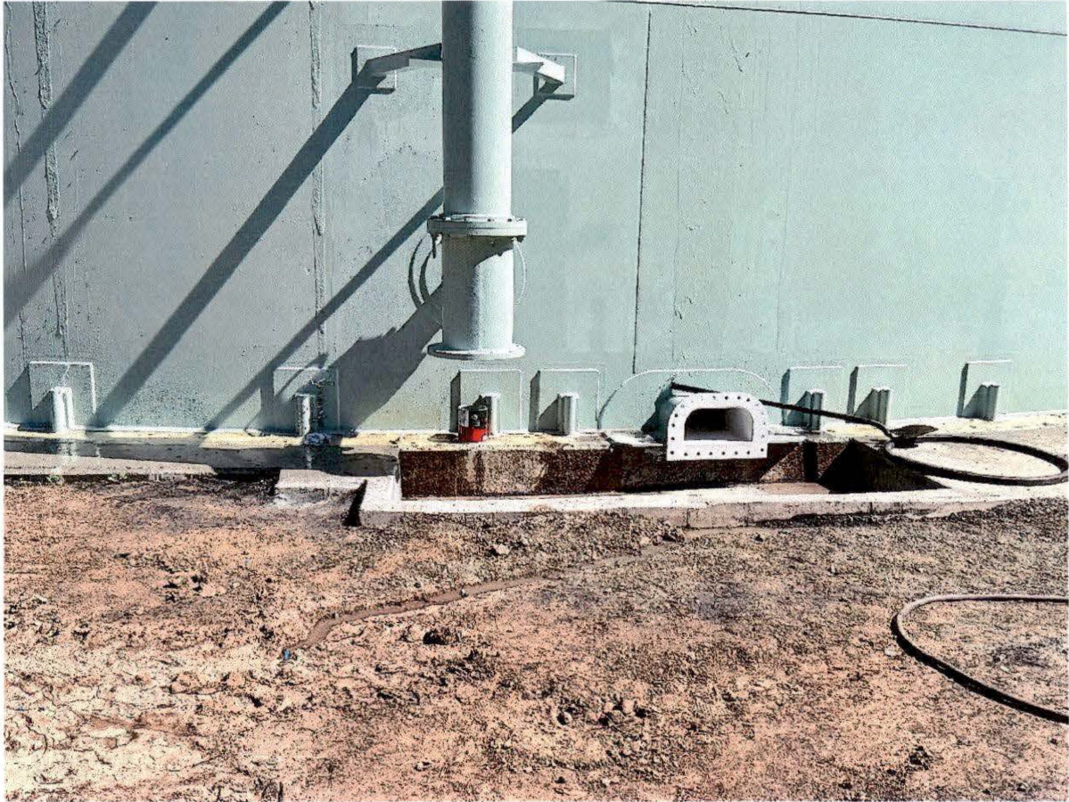
June 10, 2026 – Overflow and flush cleanout – Final coat
