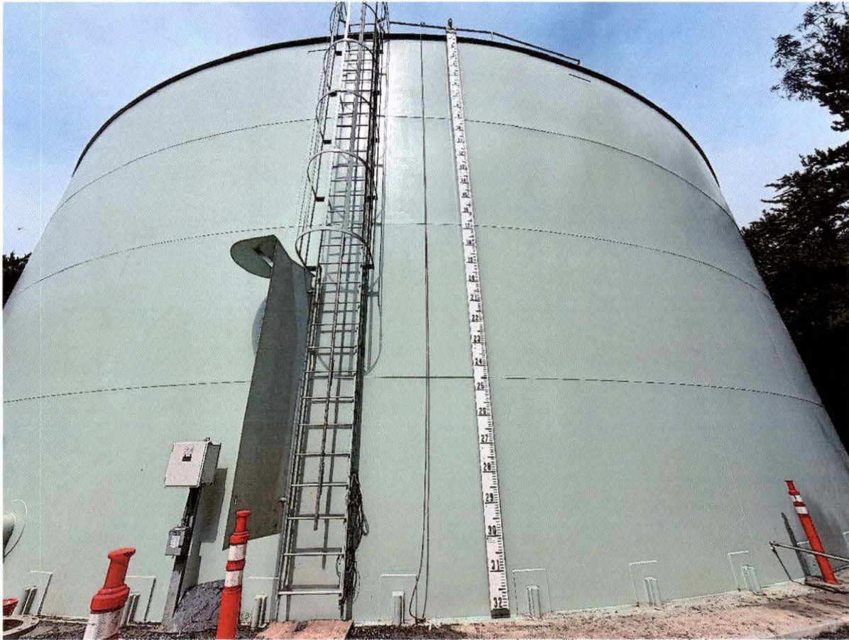
June 12, 2026 – New level indicator in place
