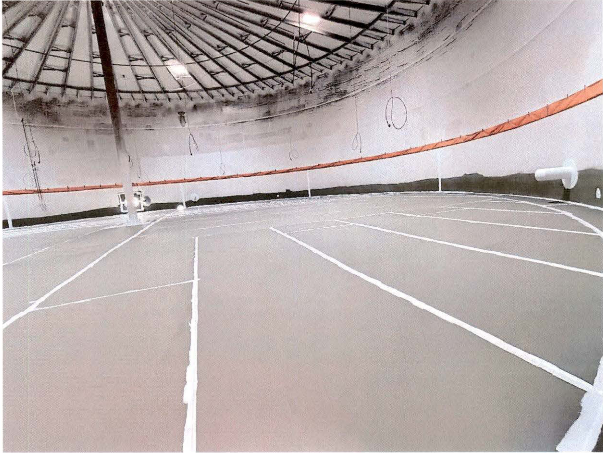
June 2, 2026 –Interior coating – Stripe Coat
