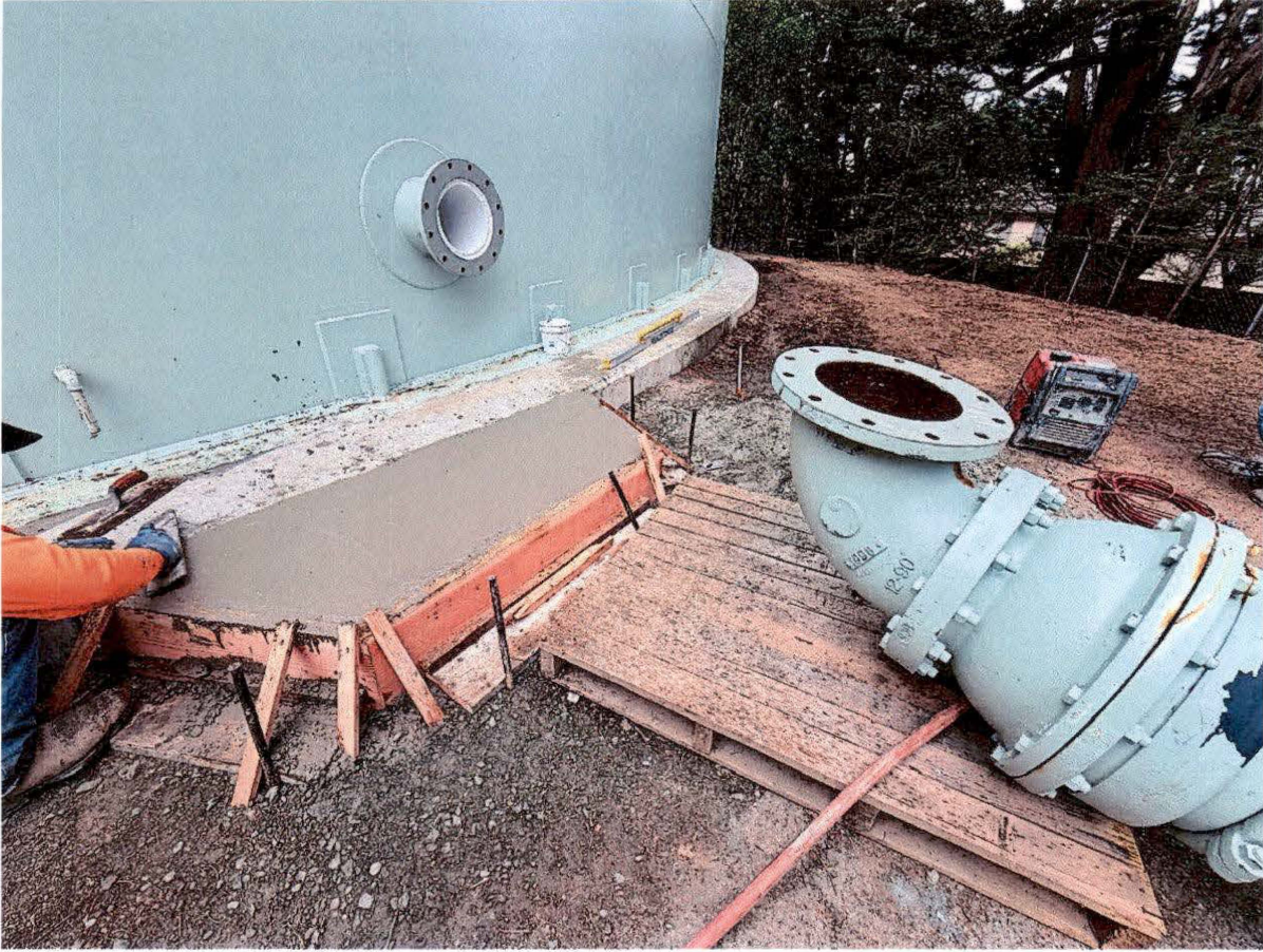
June 18, 2026 – Concrete pad placement
